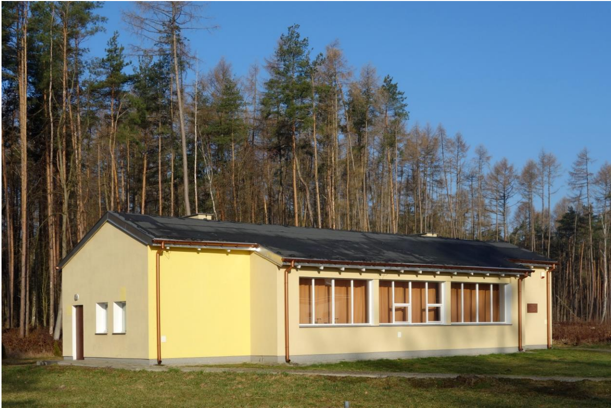
Fig. 2. Belsk Observatory – Absolute House (photo from the archives of the Central Geophysical Observatory at Belsk).
