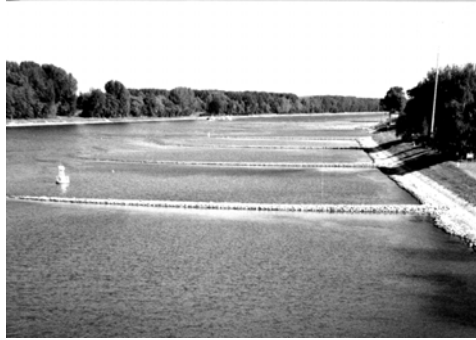
Fig. 4. Downstream view of a groin regulated river reach at low water conditions (river Rhine near Karlsruhe at km 362).
