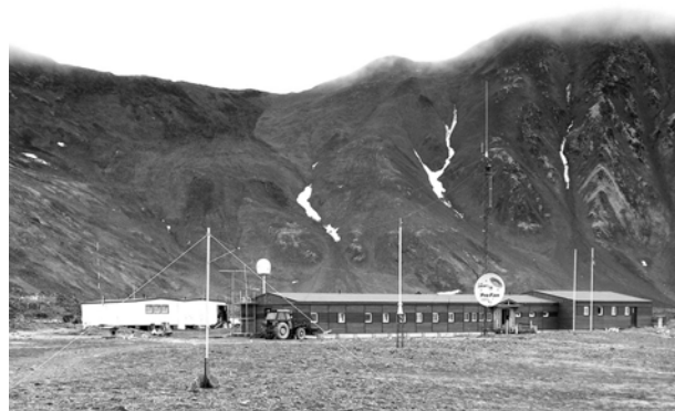
Fig. 11. The Polish Polar Station Hornsund, Spitsbergen – main building.
