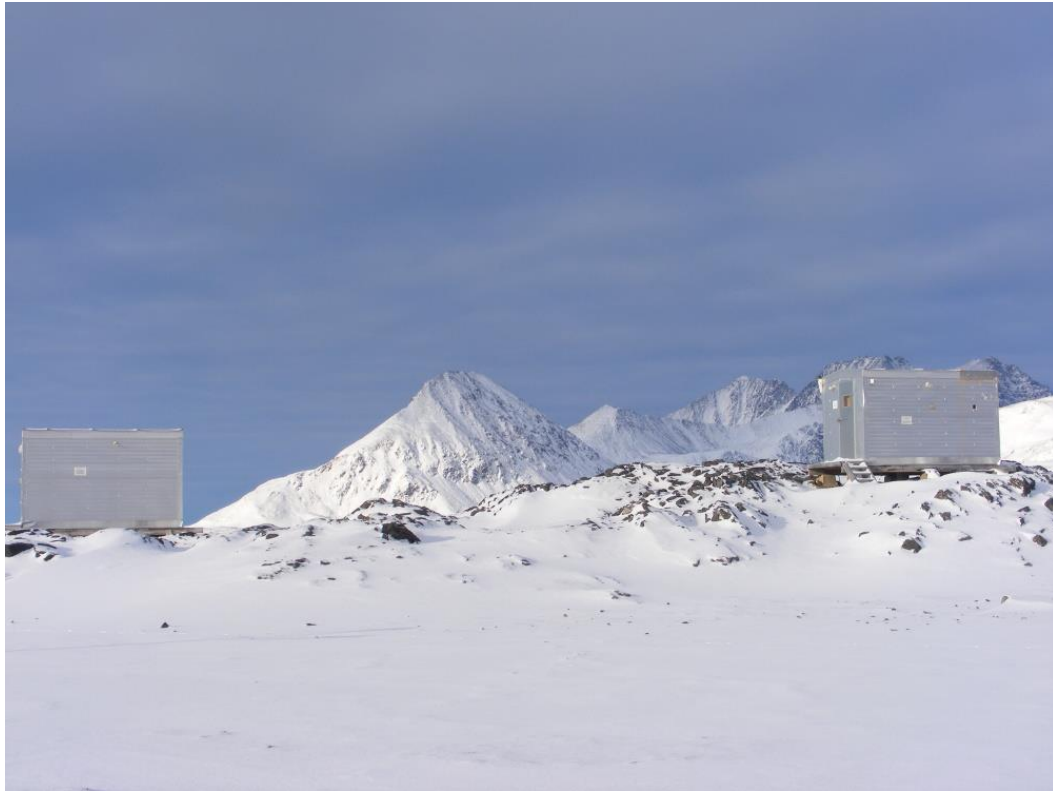
Fig. 4. The Variometer House (left) and the Absolute House (right) in PSP Hornsund, Spitsbergen.
