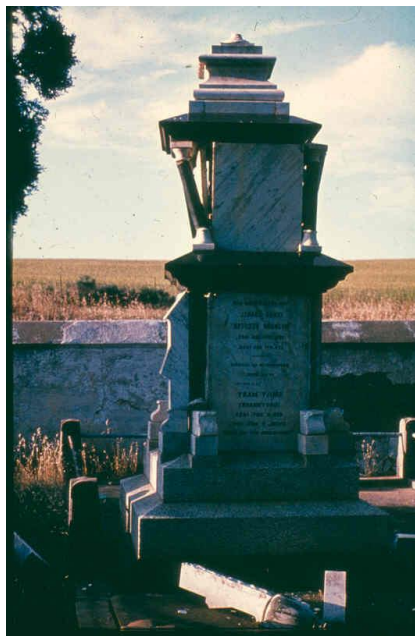
Fot. 4. Contemporary photo of the deformation of the monument; earthquake in Tulbagh-Ceres, South Africa, 29 September 1969 (after R. Teisseyre's Master Lecture).
