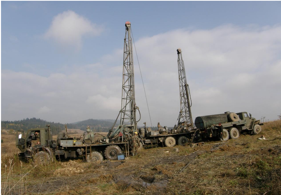
Fig. 30. Drilling works at one of the shooting points in the Carpathians (Ukraine), on the PANCAKE profile, 2008.
