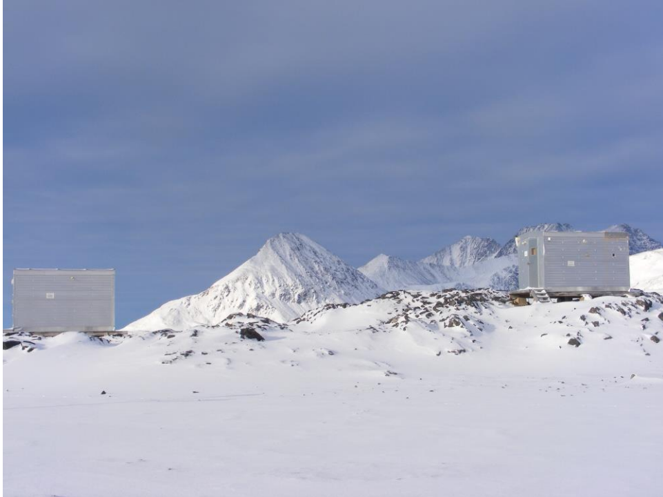
Fig. 5. The Variometer House (left) and the Absolute House (right) in PSP Hornsund, Spitsbergen.
